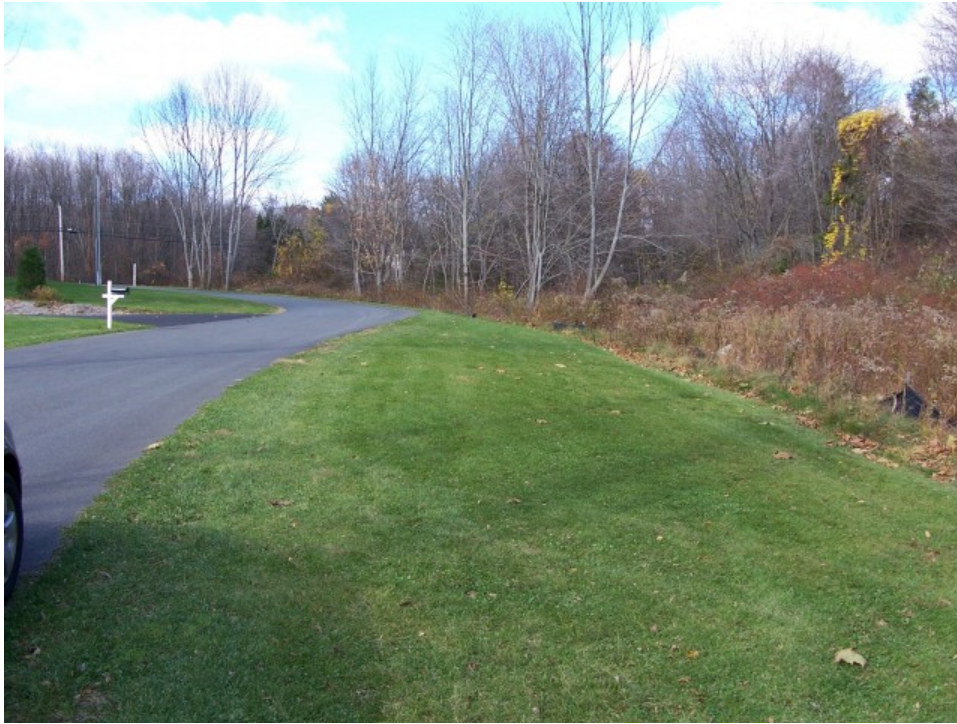
Figure 7.18.1 - Grass Filter Strip (Trinkaus Engineering, LLC - 2000)
