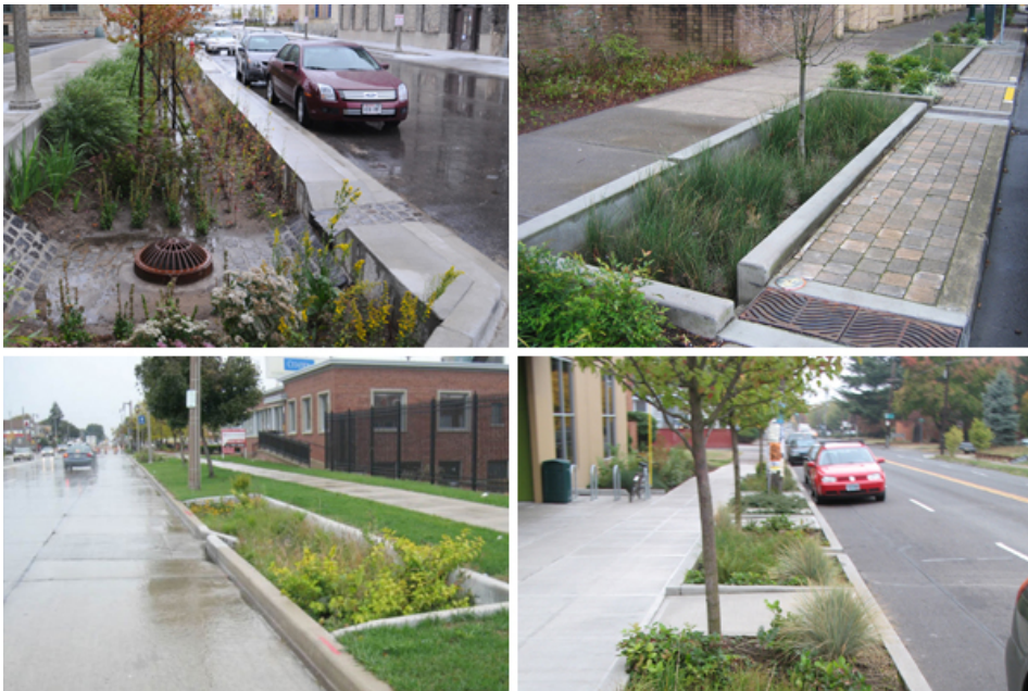
Figure 3.6.1 – LISD Street Bioretention system
