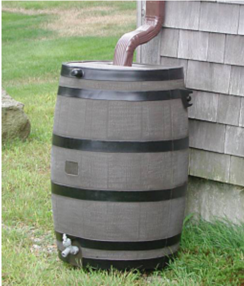
Figure 5.06.1 – Rain Barrel
