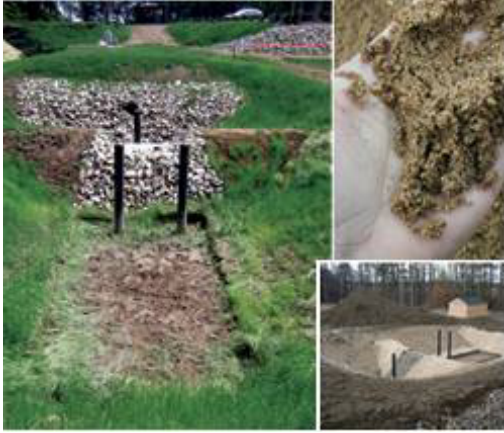
Figure 5.01.3 – Surface Sand Filter (UNHSC)
