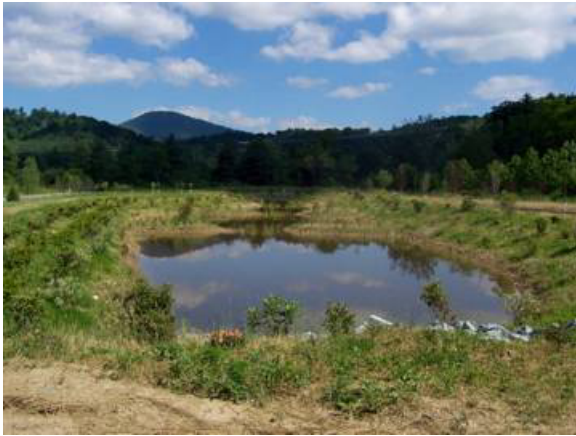
Figure 5.03.1 – Wet Extended Detention Pond (NCSU)
