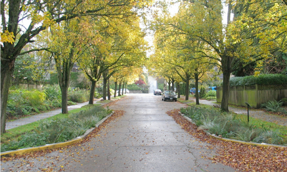
Figure 3.6.2 – LID Curb Extension Bioretention System (City of Portland, OR)
