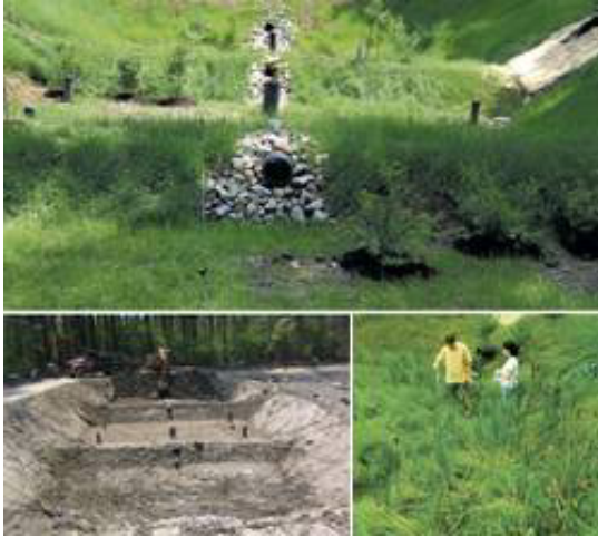
Figure 5.02.2 – Subsurface Gravel Wetlands (UNHSC)
