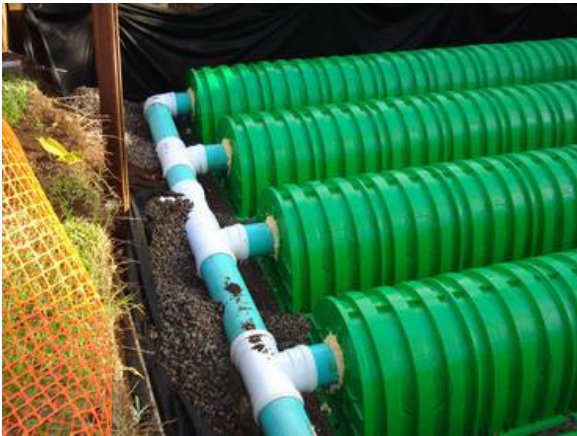
Figure 5.01.6 – Infiltration Chamber ( www.tritonsws.com/Images/case-studies )
