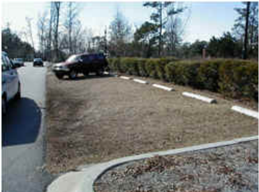
Parking Lot with Porous Surface
