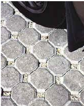
Concrete Paver Driveway
