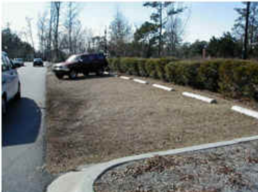
Parking Lot with Porous Surface
