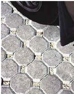
Concrete Paver Driveway
